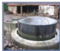
Rural Energy Systems
